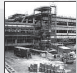
Academic Core Under Construction in 1982
